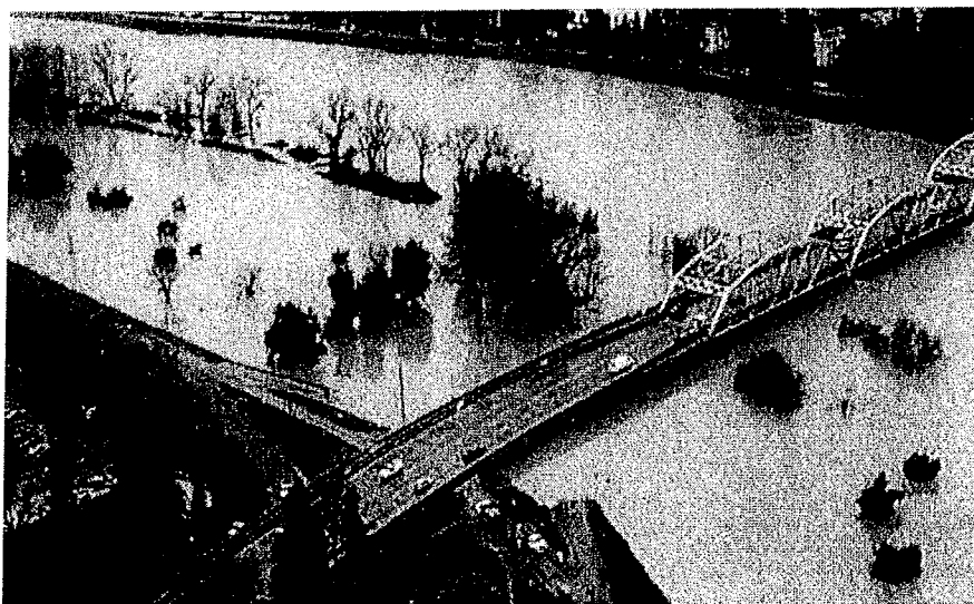
H Street Bridge during the 1986 flood event.
